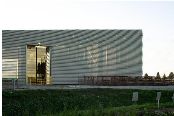
Office KGDVS, Drying hall, Hulshout, België, 2013
